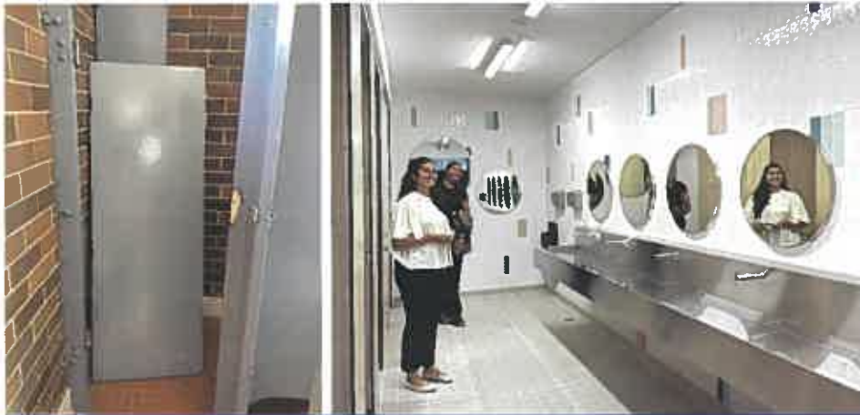
Concord High School's toilets (pictured left, before the upgrade) dated from the 1980s and had clear maintenance issues. New toilet facilities (right) were built with funding from a Community Building Partnership program grant, secured by the school's P&C Association.
